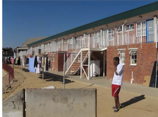
An apartheid hostel converted into affordable rooms to rent, with internal ablutions and free individual access
